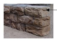
**Step 4**: Install the third course of blocks. Place a full end block on top of the half block on the second course. Continue placing wall blocks making slight adjustments as needed so that the edge of the blocks fit tightly and blocks stagger the joints on the course below. Adhere each block to the blocks below with a quality concrete adhesive. Note: You will need 2 full ends and wall blocks for the 64" wall or 2 full ends and 10 wall blocks for the 112" wall.
