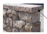
**Step 5**: Install the caps. The first cap should be placed at one end of the wall leaving an approximately 1" overhang on both sides and the end. Adhered each cap to the blocks below with a quality concrete adhesive. Note: You will need 3 full and one half cap for the 64" wall or 6 caps for the 112" wall.
