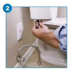
Connect the t-valve to the fill valve under your toilet
