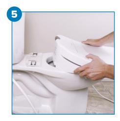
Attach the Swash to the mounting plate
