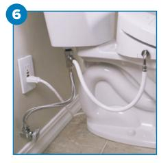
Connect the bidet hose to the Swash, turn on the water, plug in the power cord
