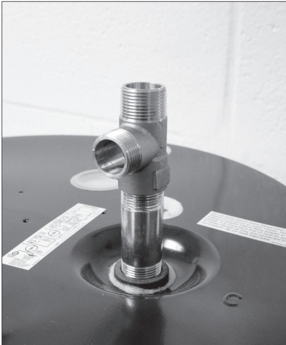
4. Apply sealing tape to the male threads of the mixing valve and tee. Check the installation orientation of both to ensure that the connection of the flexible hose can be allowed.
