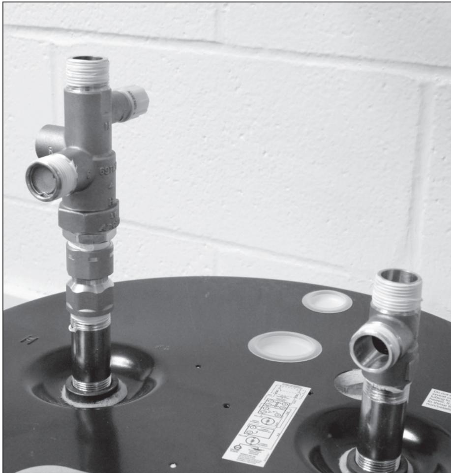
5. Connect the flexible hose from the mixing valve to the tee as shown below.
