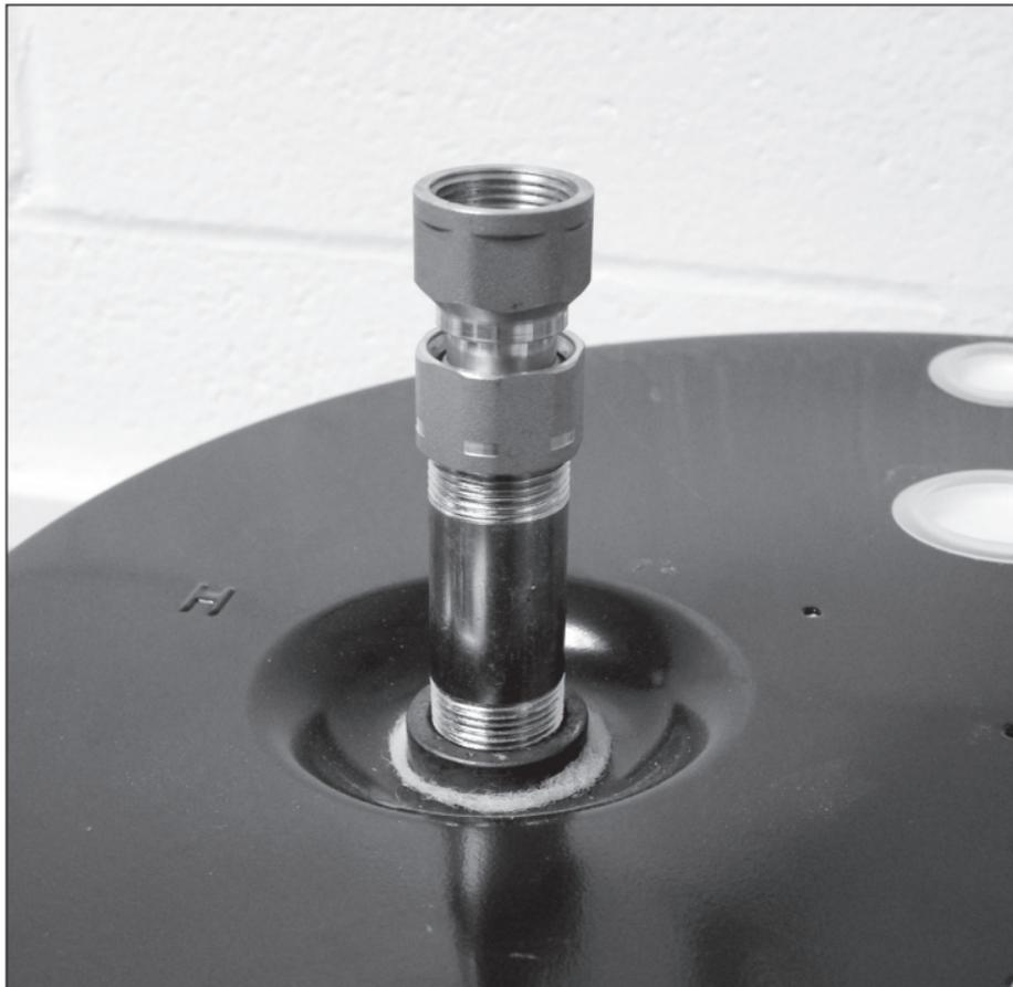
2. Attach the mixing valve to the union fitting as shown below.
