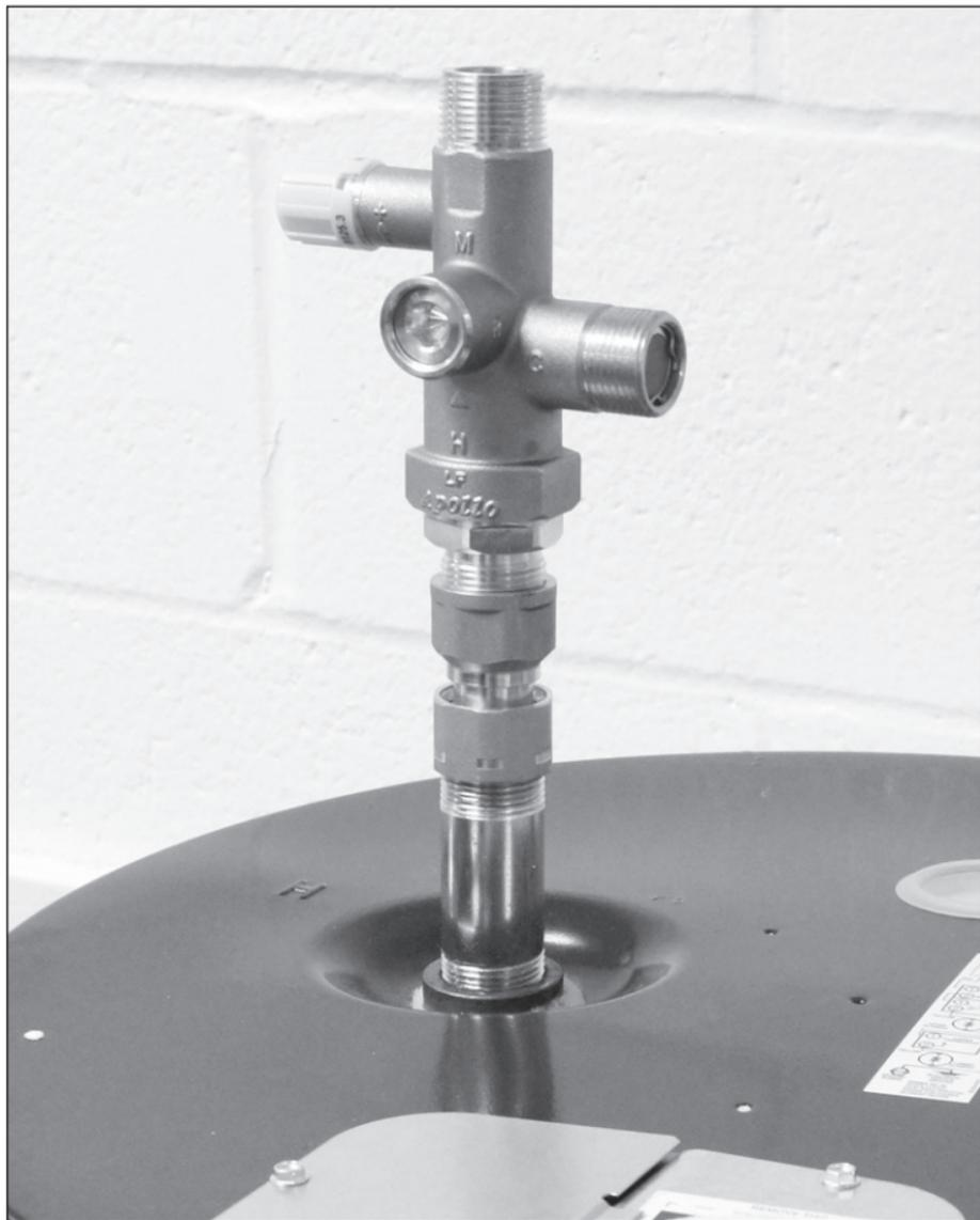
3. Connect the tee to the cold water inlet of the water heater.
