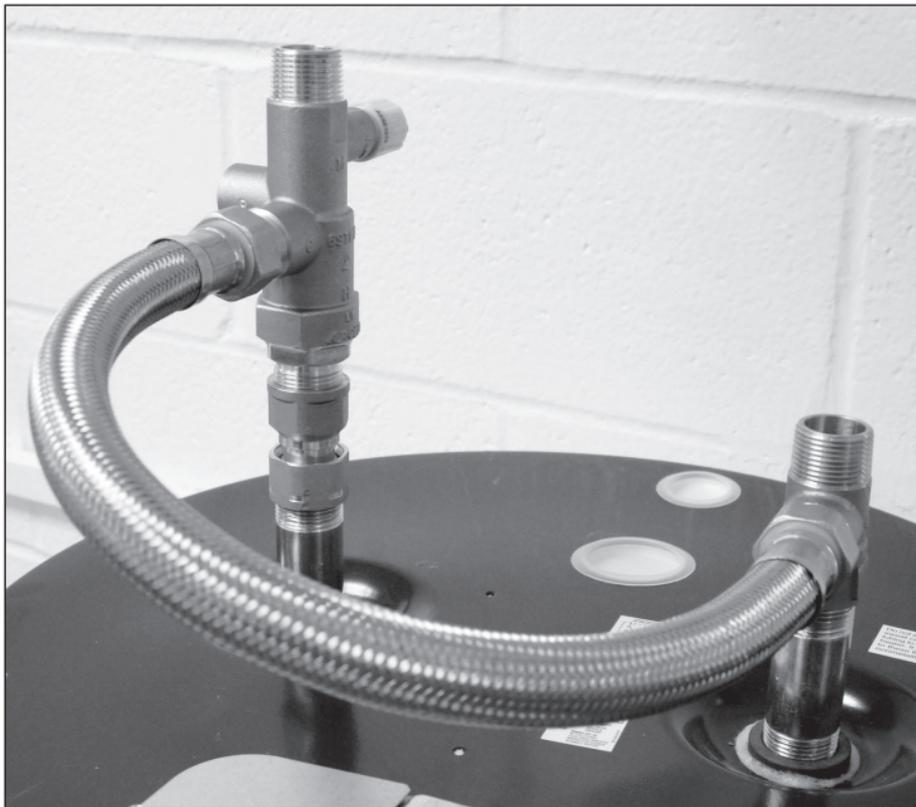
6. Connect the system's cold water inlet supply hose to the tee and the hot water outlet supply hose to the mixing valve.
