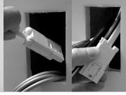
Drop or wall-fish audio/video cables within wall BEF<u>ORE</u> PowerConnect cable
