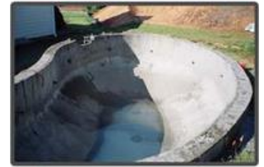
1. Prepare the Surface
