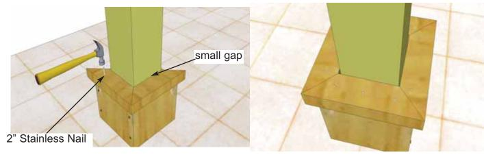
**26.** Position **Post Skirting Caps - 1** 1/2" x 2 1/2" x 10 5/8" (Part L) on top of skirting unit and against post. Do a dry run first to confirm fit. There will be a small gap between post and inside of cap. Attach caps down into skirting tops with 3 - 2 1/2" **Stainless Steel Finishing Nails** per piece. Complete remaining post skirtings.
