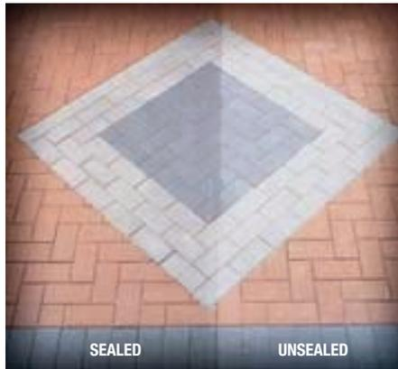
One way to moderate the rate of color change is by cleaning and sealing the surface of the concrete pavers. Besides enhancing their color, sealers can prevent dirt from lodging in the surface.
