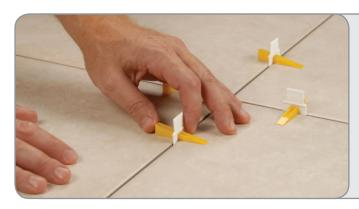
**LEVEL:** Anchor adjusts to the tiles so they remain level throughout the installation
