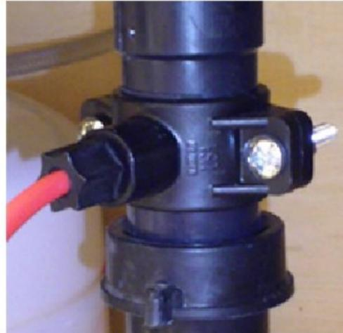
Fig. 5 Drain saddle
